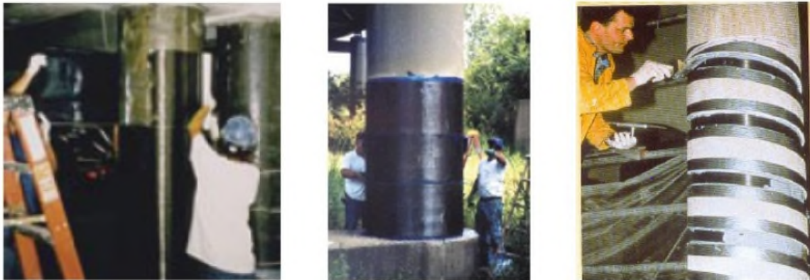
Figure II.23 : Stratification au contact (WBAC 2003) [57]
