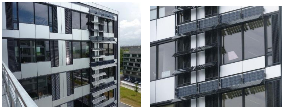
Figure IV. 24: brise-soleils et panneaux photovoltaïque poly cristallins en bardage
