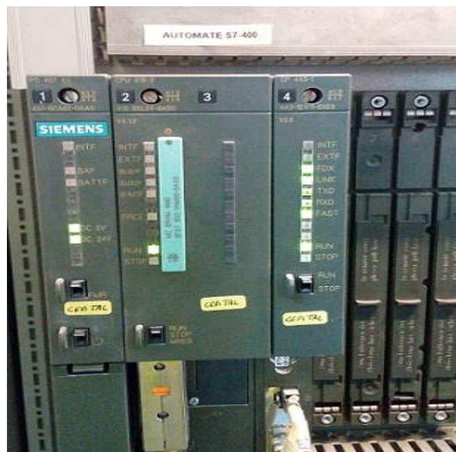
Figure II.7.1 Automate programmable S7 400
