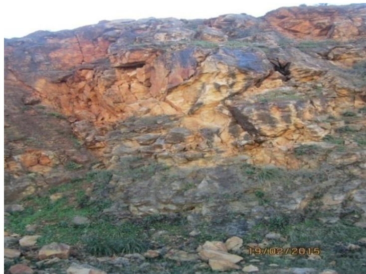
Figure IV. 5: Chute des pierres
