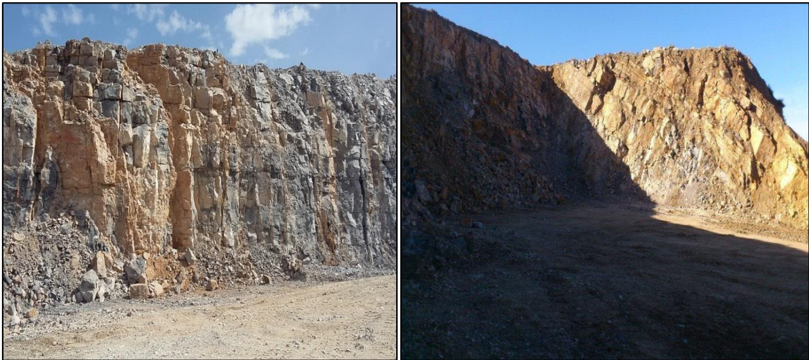
Figure III.1: Différentes conditions de fracturation in-situ (Ain El-Kebira, 2016)
