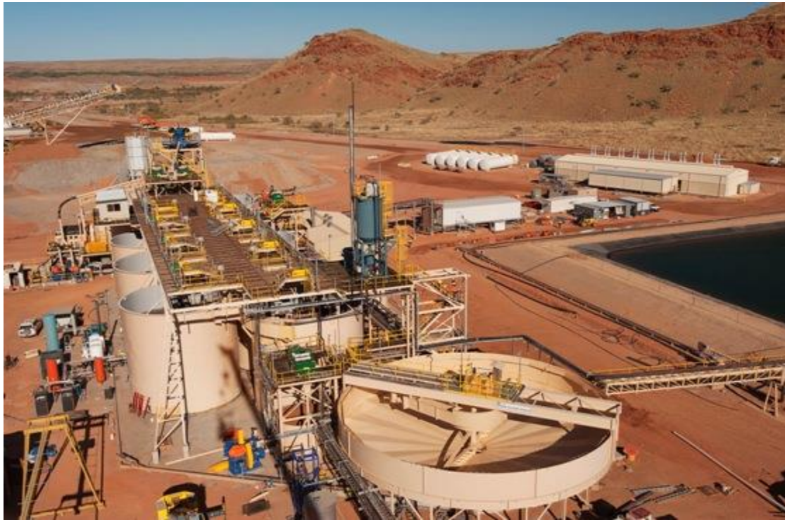
Figure II.5: Le circuit CIL. [32]
