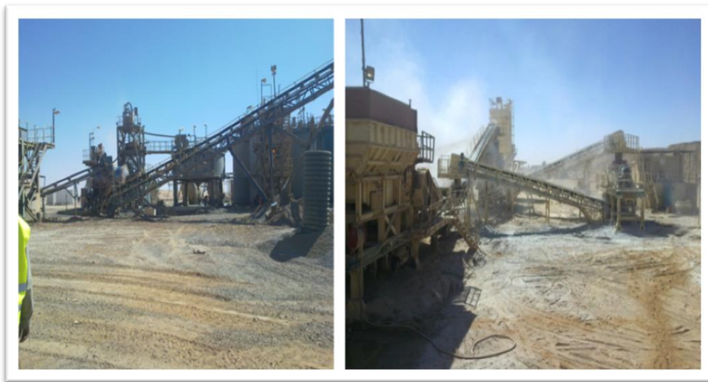
Figure II.7: Station de concassage. [Source : Photo prise]
