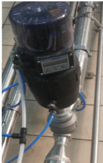
**Figure III.26:** Vanne modulante burkert type 8630
