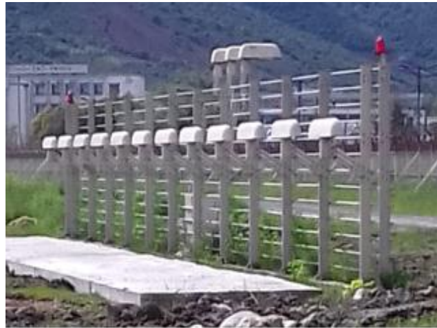
Figure (III. 6) : Antenne du localizer.
