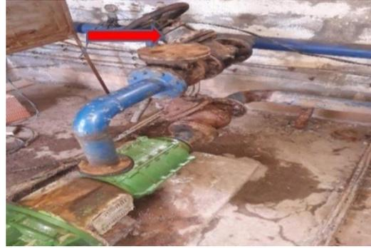
Figure 15: Vanne corrodé
