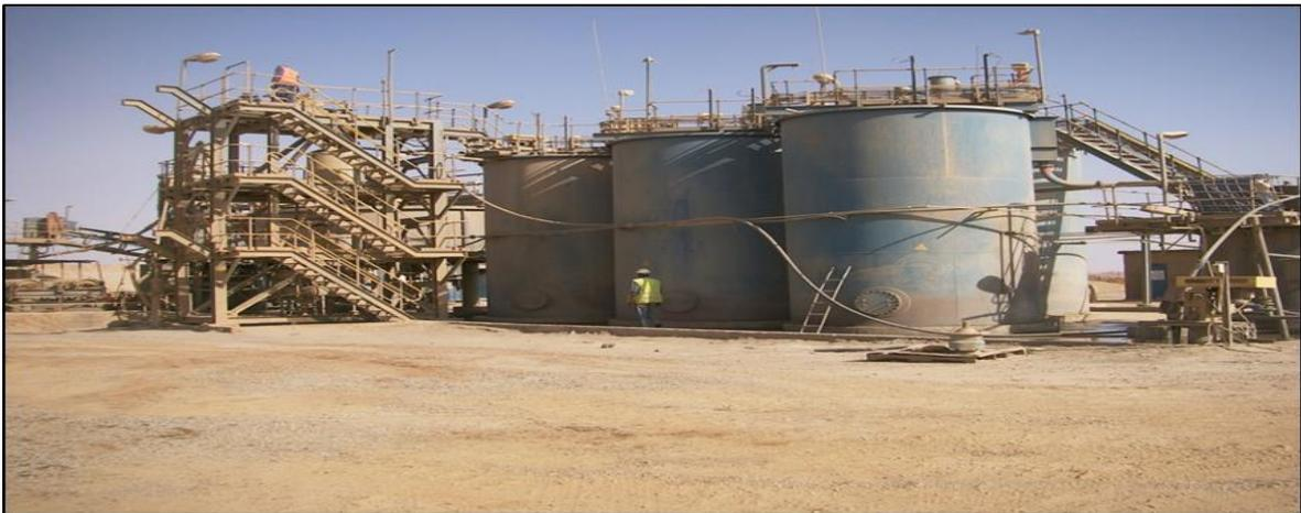
**Figure I.11 :** Cuves de lixiviation (photo prise).
