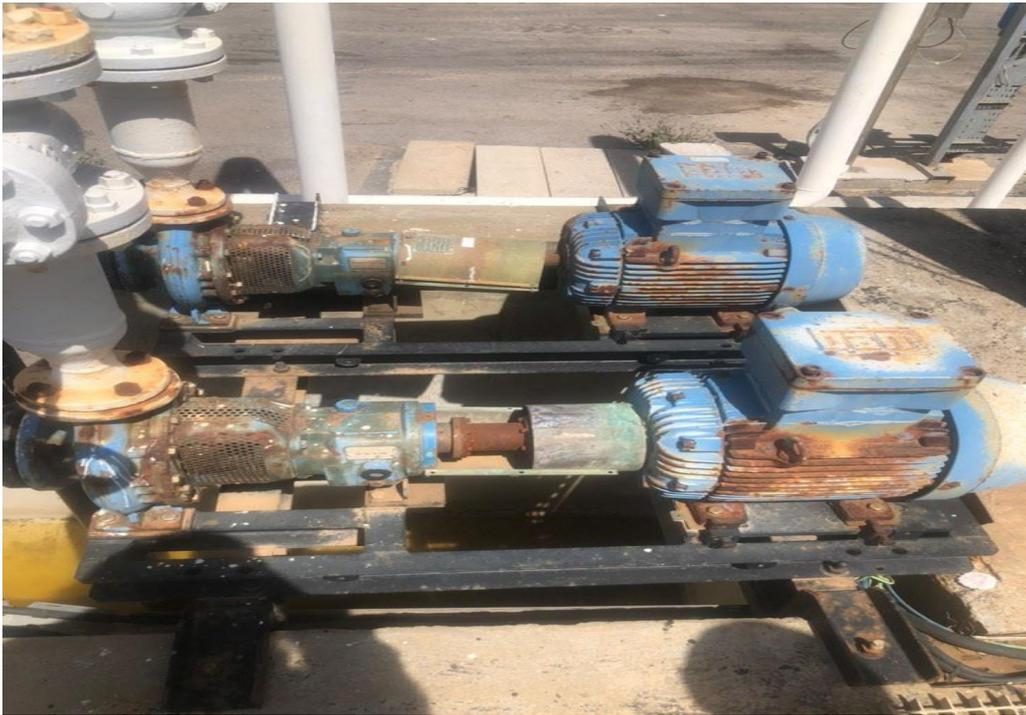
**Figure I-6 :** pompes centrifuges
