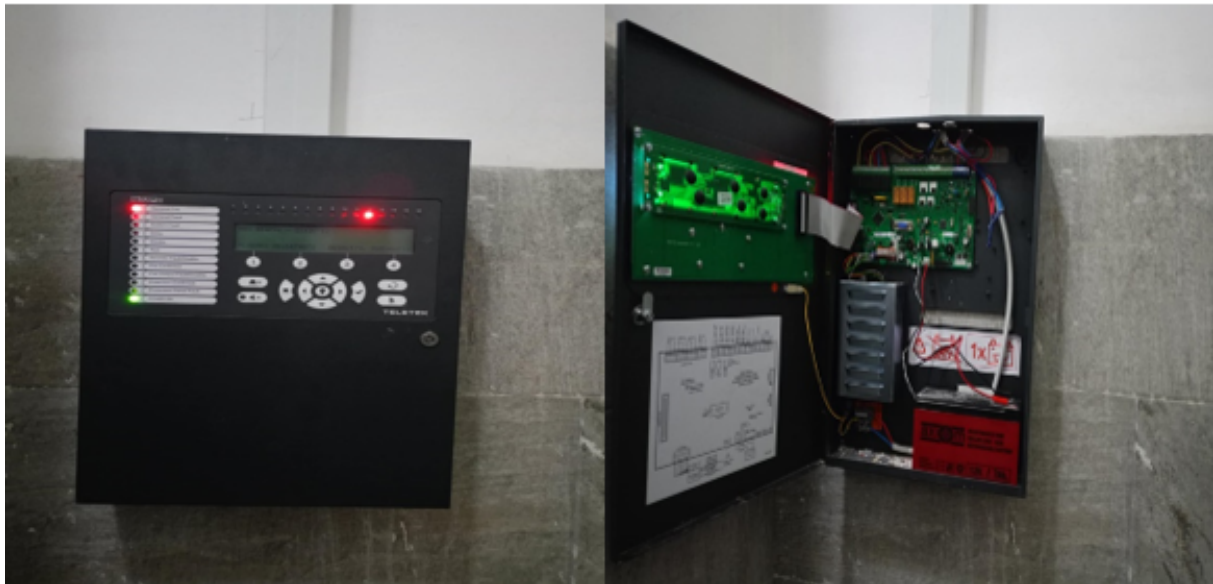
FIGURE II.7 – Centrale désenfumage TELETEK [12].
