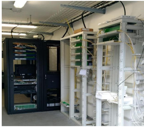
Figure 2.13: The Optical Distribution Node.
