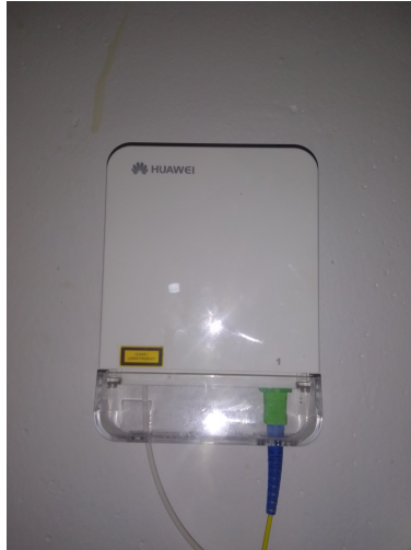
Figure 2.19: The Optical Termination outlet.
