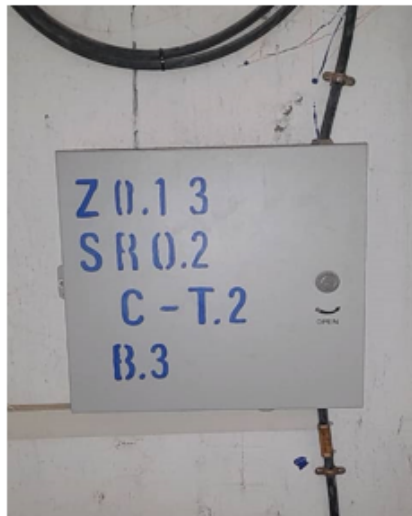
Figure 2.17: indoor Optical Branching Point.
