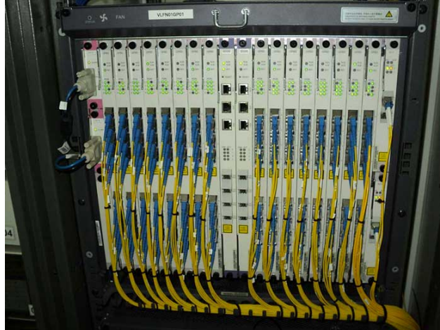
Figure 2.14: Optical line termination.
