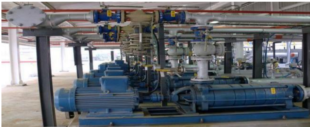
Figure III-4 Pompes GPL.
