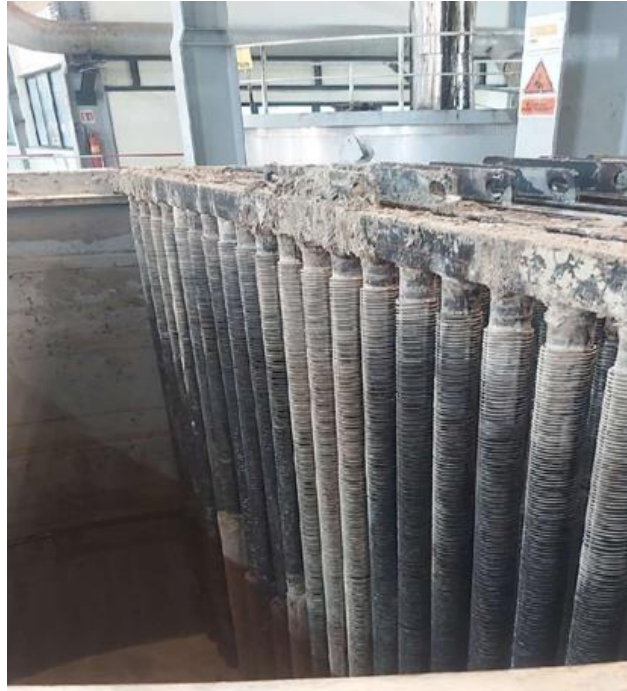
Figure I.6: Rampes supportant des bougies
