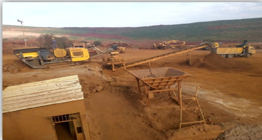
Figure III.7: Station de concassage de la mine de Rouina.
