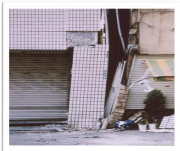
**Figure I.10.** Joint parasismique insuffisant
