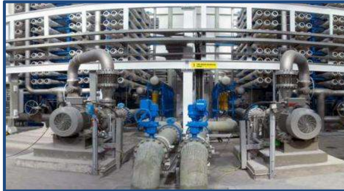
Figure IV.13 : Pompes BOOSTER
