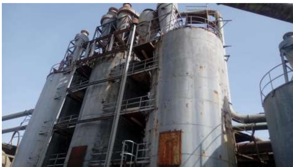
Figure III. 5. Silo de stockage.
