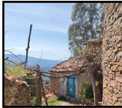
FIGURE 29 : FACADE IMAGE OF KABYLE HOUSE
