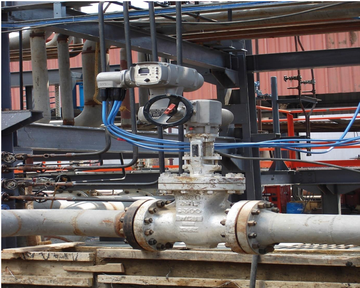
Figure I.11 : Vanne TOR.
